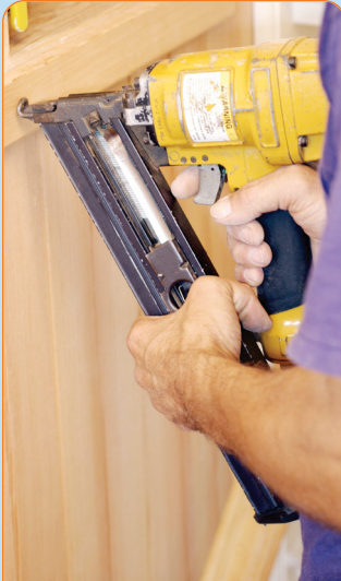
Repeated use of tools that vibrate the hand and wrist can lead to RMIs.
