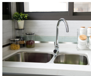
Sinks and faucets
